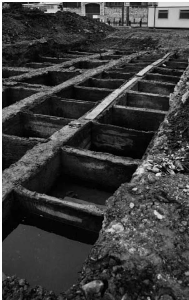
Fig 5. Site of Stanley's Tan Yard during excavations in 2002
