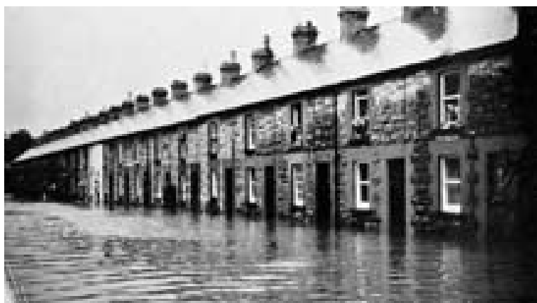
The Mill Row in flood
