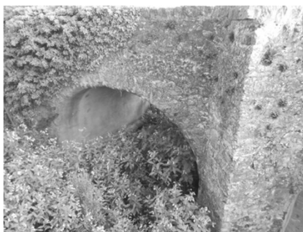
Fig. 10. The first two eastern arches are silted up and
