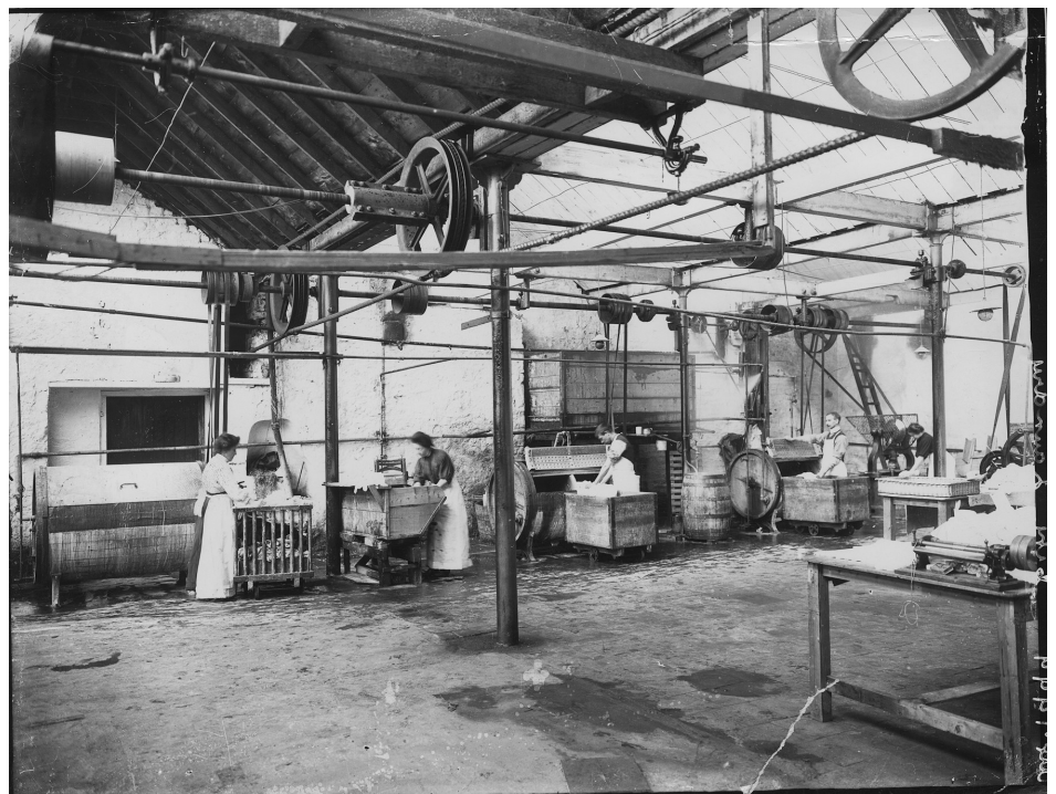
The Washing Room, Armagh City Steam Laundry c1915. Two of the cylinder type washing machines are being loaded by men but the majority of workers were women. The drive shafts and belts that operate the machinery were inherited from the weaving factory that occupied the site before 1903.
