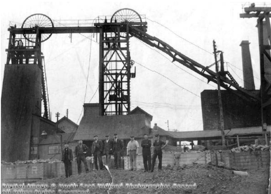
Cinderhill Colliery showing the twin shafts that provided ventilation in the mine, a fire was lit at the bottom of one of the shafts and the rising hot air pulled fresh air down the other shaft to provide ventilation. The mine remained in operation until the mid 1980s. I am grateful to Picture the Past ( www.picturethepast.org.uk ) for kind permission to use this image of Cinderhill Colliery.
