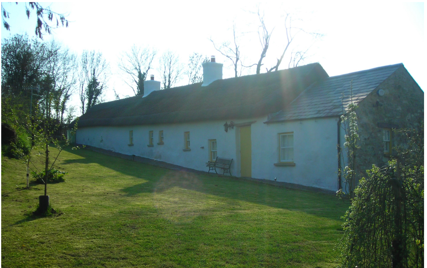
Fig.14 showing the back elevation after the completion of the restoration project. Fig 15 showing the front elevation can be seen on the back cover. (Photos courtesy of Eddie O'Neill)
