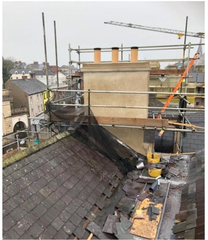
View of the roof valley mended to stop leaks
